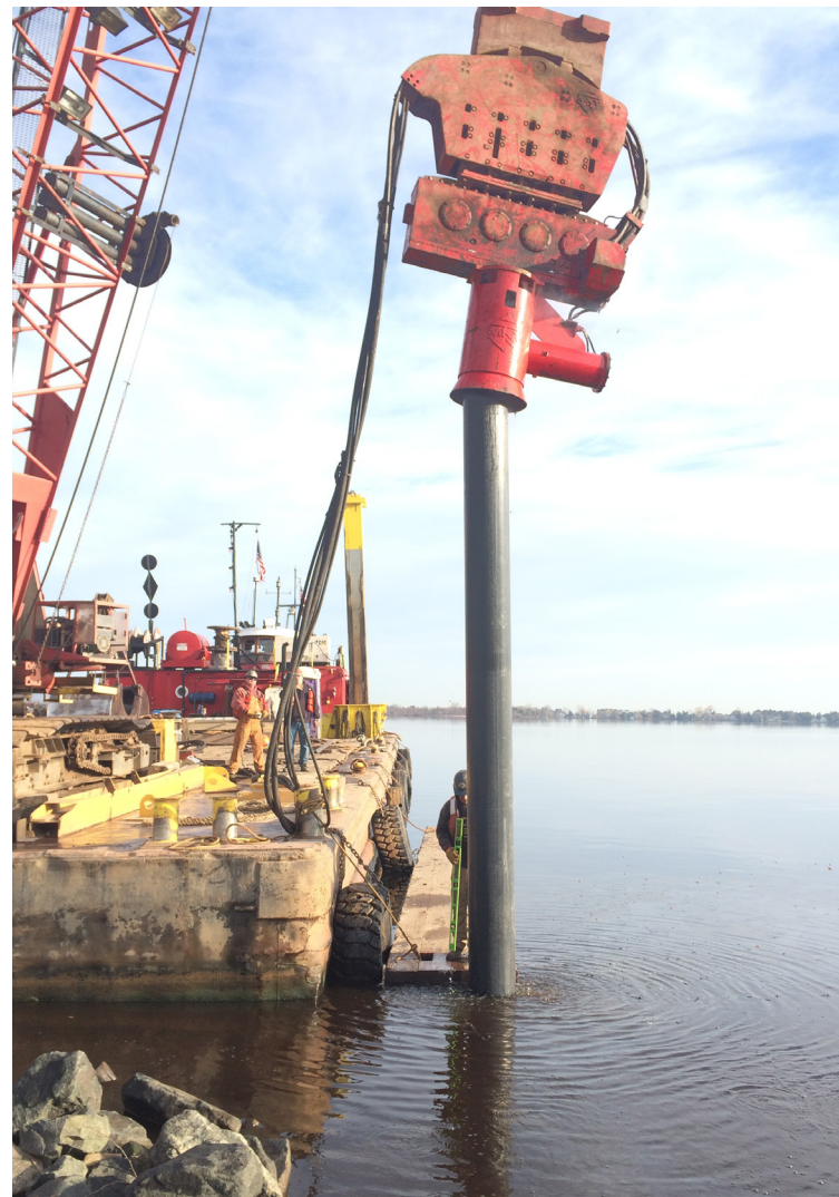
Figure 1: Test Pile Installation November 2015
