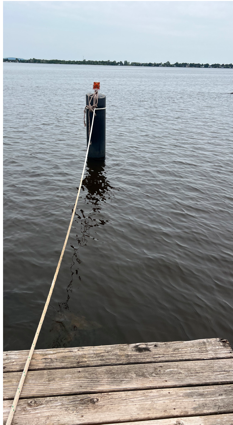
Figure 4: Test Pile in July 2023
